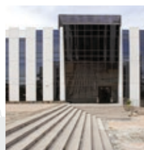
MADRID GLOBOMEDIA PROJECT BY BNB PROJECT
